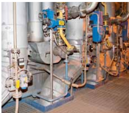
REBOX® HLL installed in a furnace
