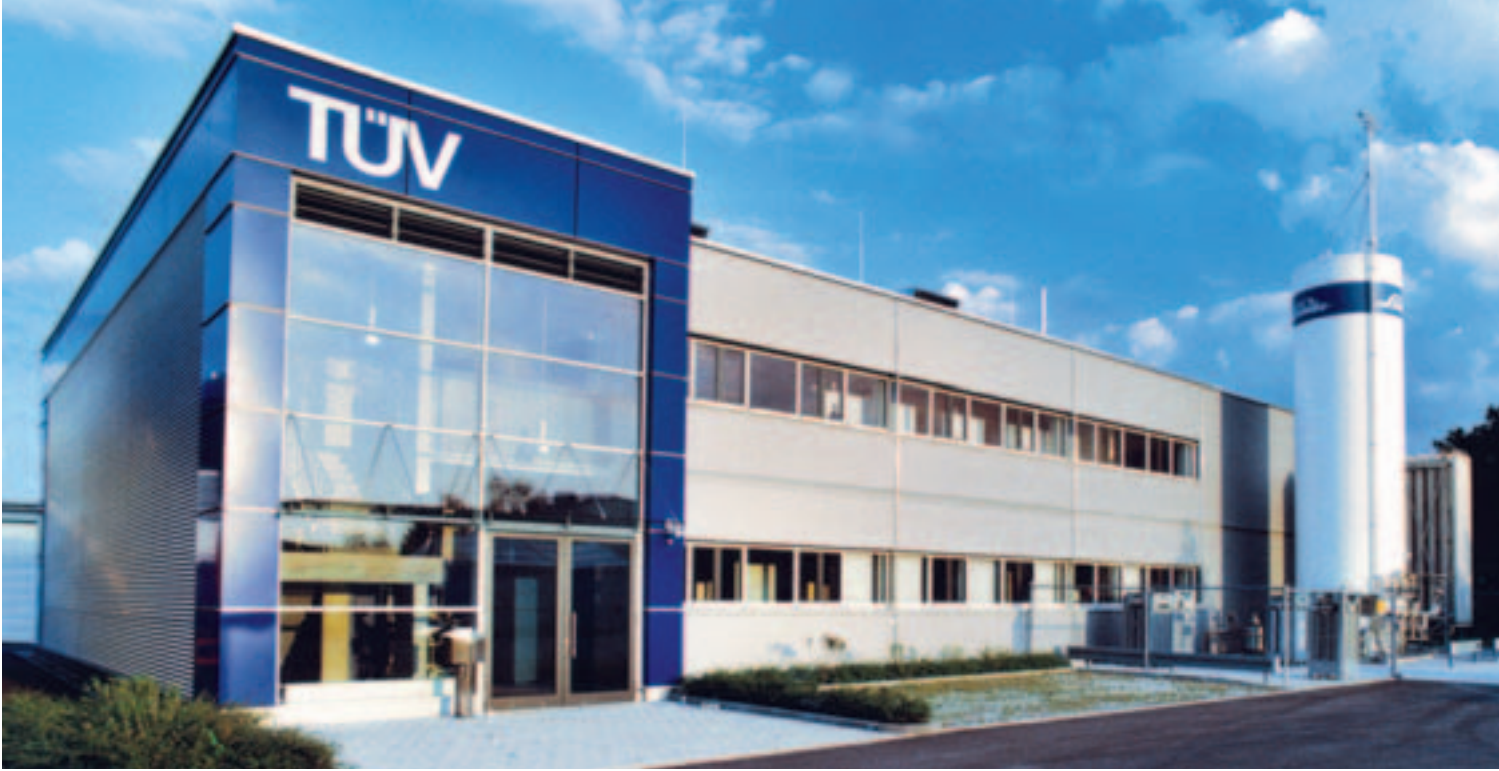
The first HAT reference project, under way since November 2002: the hydrogen engine and drive chain test center in Garching, near Munich.
