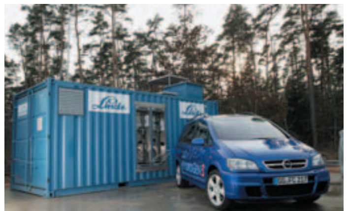
Filling a hydrogen car at a 700 bar filling station for GH 2 .
