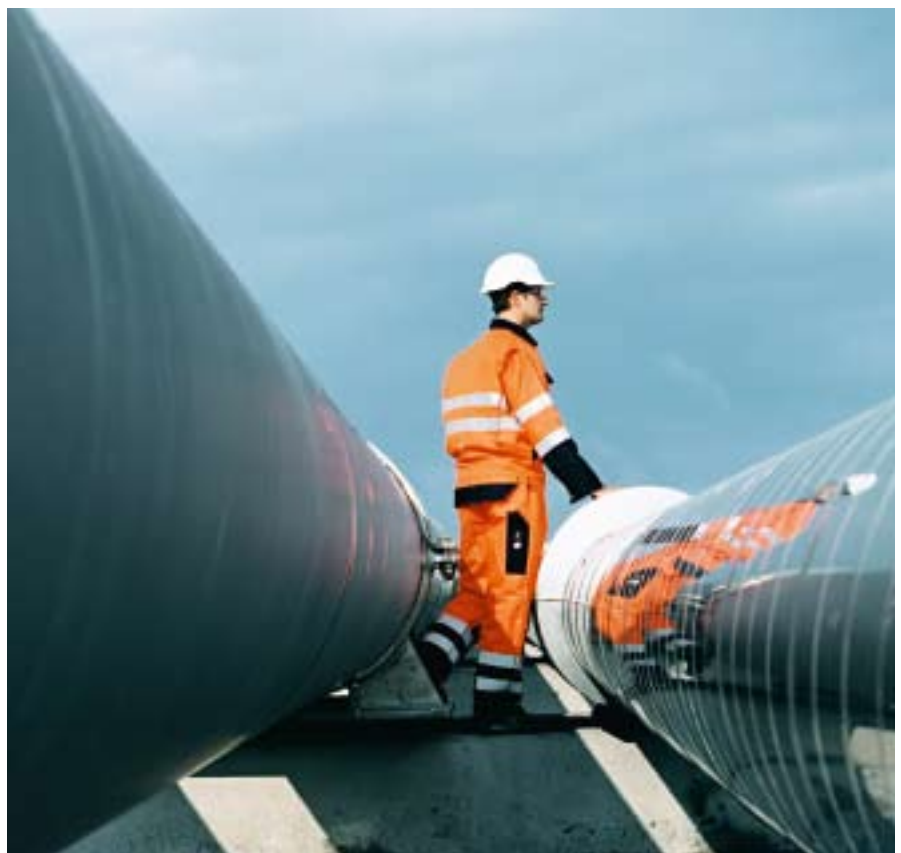
↳ (top) The world's largest air separation complex in Qatar – engineered by Linde.
