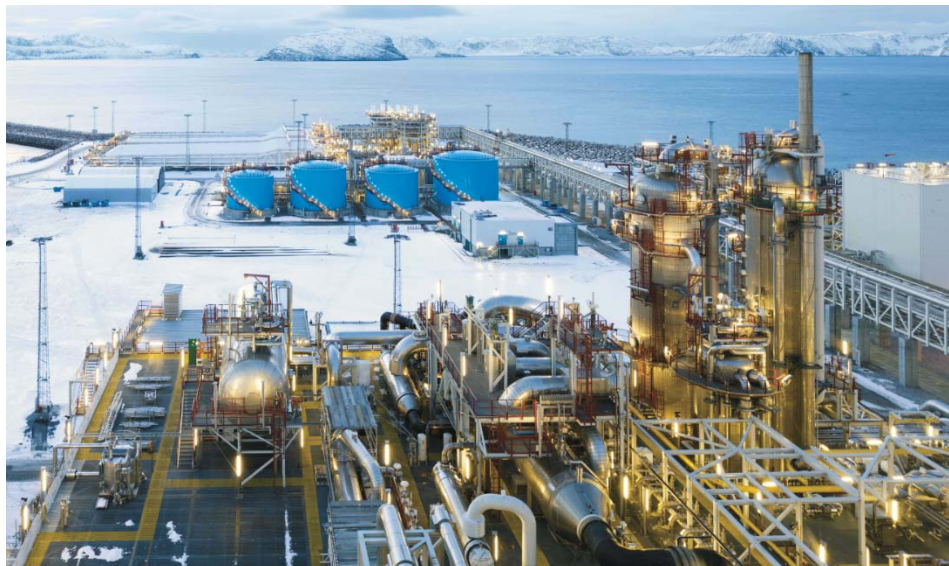
Image caption: Onshore plant for natural gas processing (© The Linde Group).
